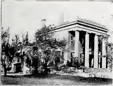
Home of Erastus Gaylord, on Woodland avenue, built 1836. Type of the classic columns then much in vogue.
